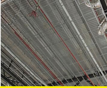
SteelMax Lightweight Ceiling System where the runners and channels form a rigid structural support for Gypsum board, Drop ceiling assemblies or Plasterboard. This cost saving ceiling system provides a structurally sound, uniformly level, benchmark framework for flush ceiling boards. All SteelMax ceiling profiles are manufactured to BS 5950
